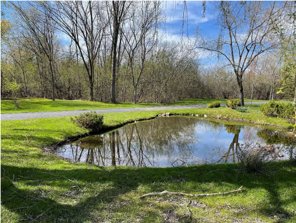
4. Pond (presumably excavated) with landscaping and culvert facing northwest.
