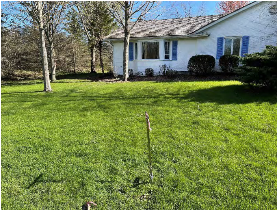
2. Data point 2UPL (Upland) facing south viewing front (north side) of residence.
